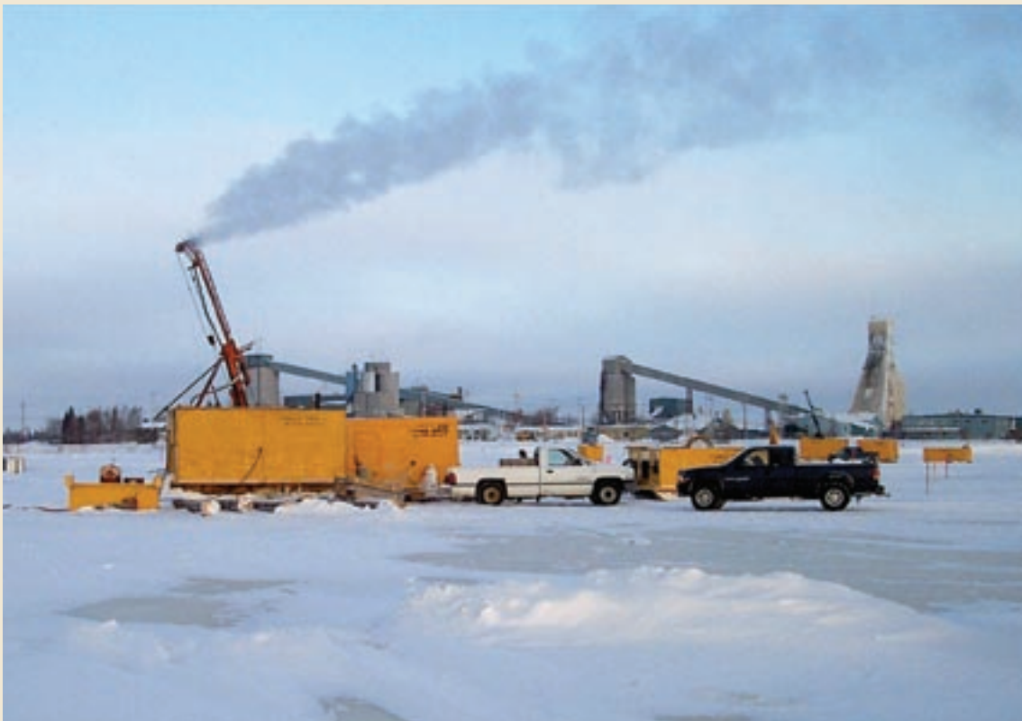
Drilling on the ice, 2003 southeast of the Kiena Shaft.
